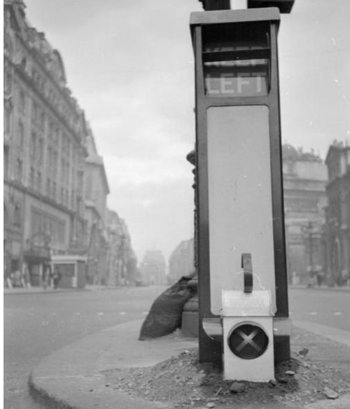
Figure 3-3. Bollard on a traffic island in London. To help prevent accidents during the blackout the bollard is painted white and has the words 'Keep Left' the top of the bollard, Imperial War Museum, D 2732, https://www.iwm.org.uk/collections/item/object/205198119 .
