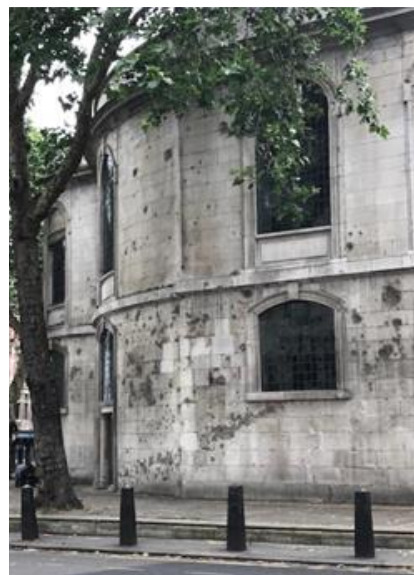
Figure 6-11. St Clement Danes preserved shrapnel damage, June 2, 2019, St Clement Danes Church. author's personal collection.
