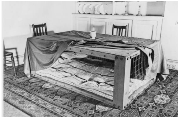
Figure 5-8. A Morrison shelter set up in a dining room, 1941, Ministry of Information Photo Division Photographer, Imperial War Museum, D 2053, https://www.iwm.org.uk/collections/item/object/205197886 .
