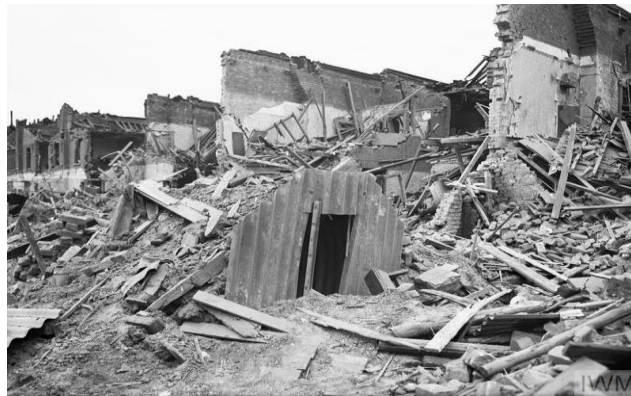
Figure 5-6. An Anderson shelter remains intact amidst destruction in Latham Street, Poplar, London during 1941, Ministry of Information Divisional Photographer, Imperial War Museum, D 5949, https://www.iwm.org.uk/collections/item/object/205198906 .
