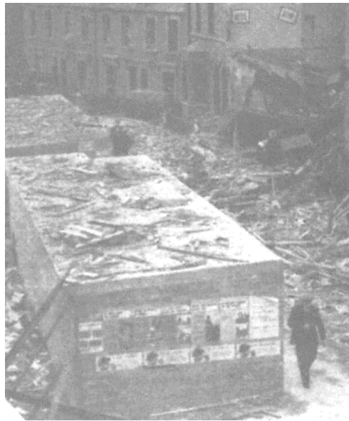
Figure 5-4. Surface shelter emerges unscathed after bombing raid, 1940, War Illustrated .
